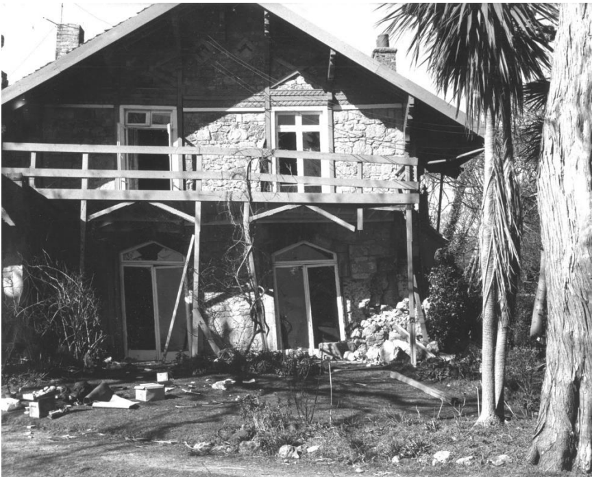
Figure 3.18.21.: 'Sandrock Spring Cottage' at Blackgang was an elegant chalet style property located to the south-east of Blackgang Chine. Coastal erosion and slope instability led to the collapse of the property and the adjacent public highway in March 1978.
