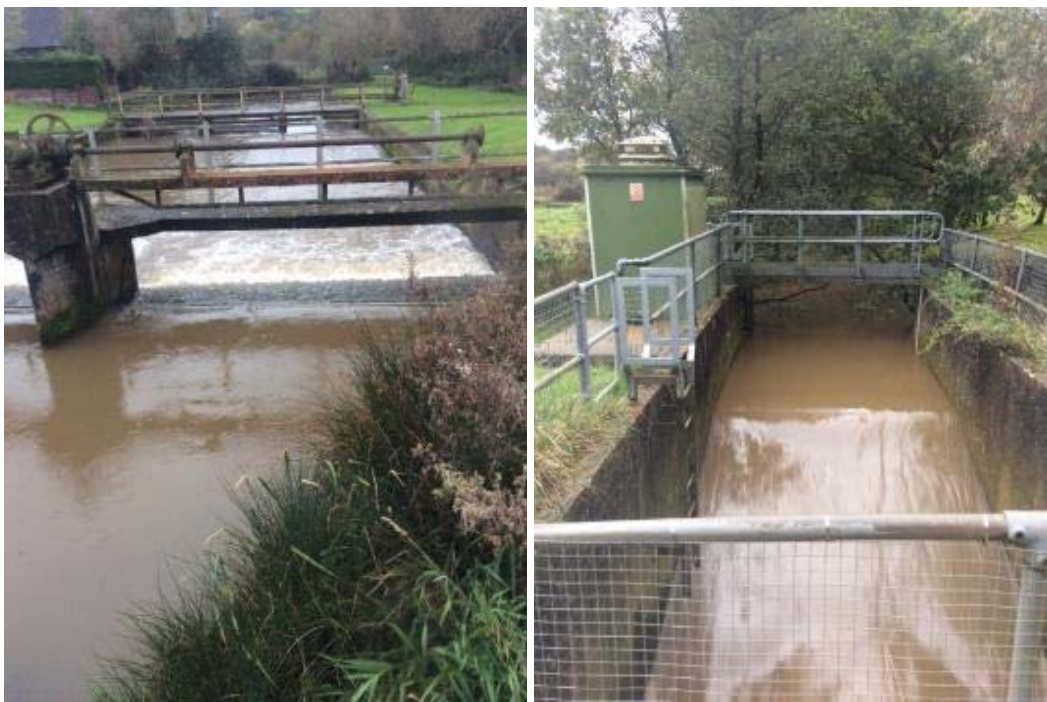
Figure 11: Example barriers to fish passage (Left - Alverstone Mill Sluice, Right - Budbridge gauging station).
